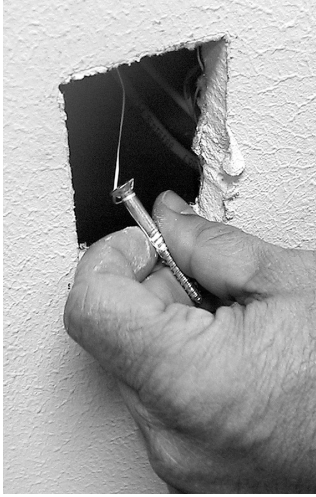
FIGURE 6-4 Dropping the cable
