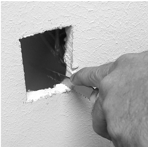
FIGURE 6-2 Cutting a hole
